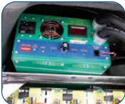
■ FIGURE 7. The inverter in the boot.
